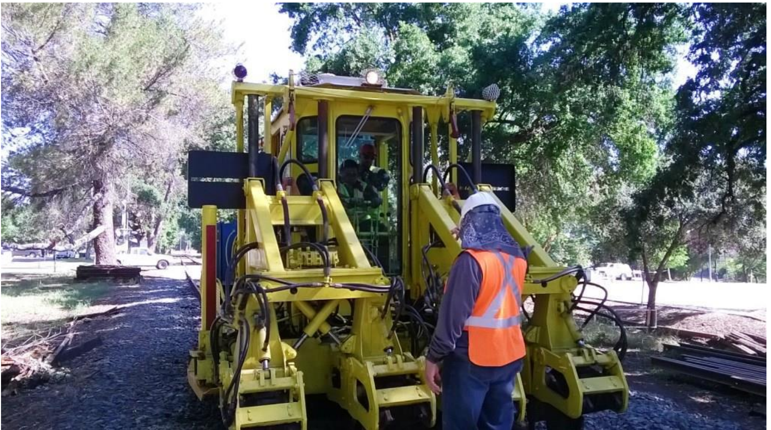
In the Tamper, Chris gives Anthony a lesson in its operation as Jose guides from the ground
