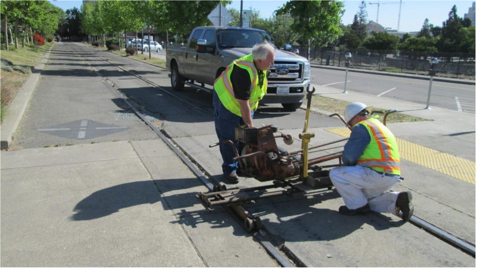
After a 32-block detour, the bolt machines finally reach the job-site. Harry and Mike H. get them started
