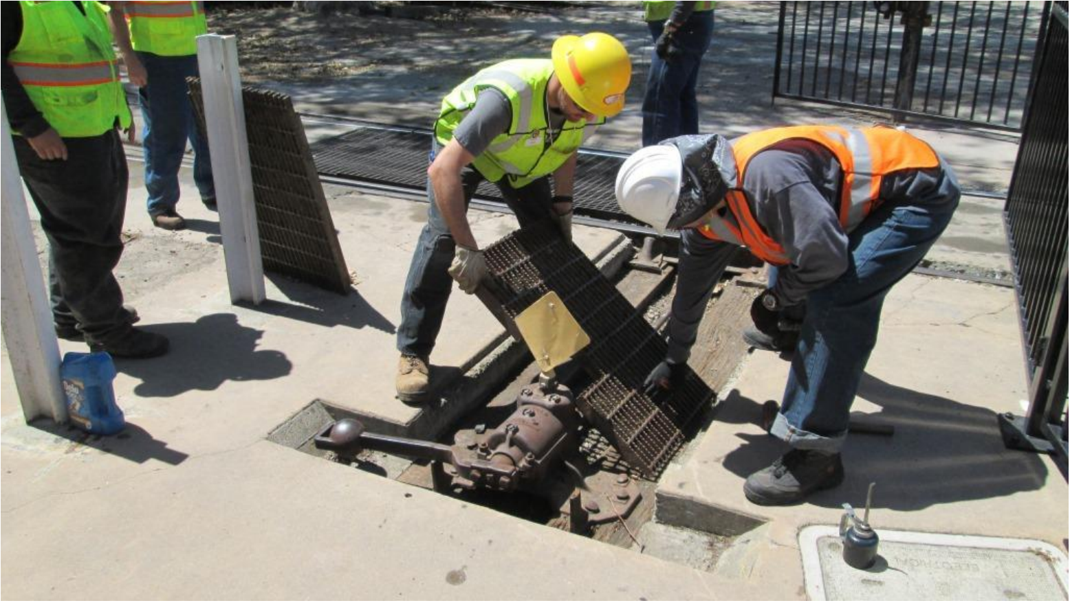
Chris and Jose replace the grating over the switch components
