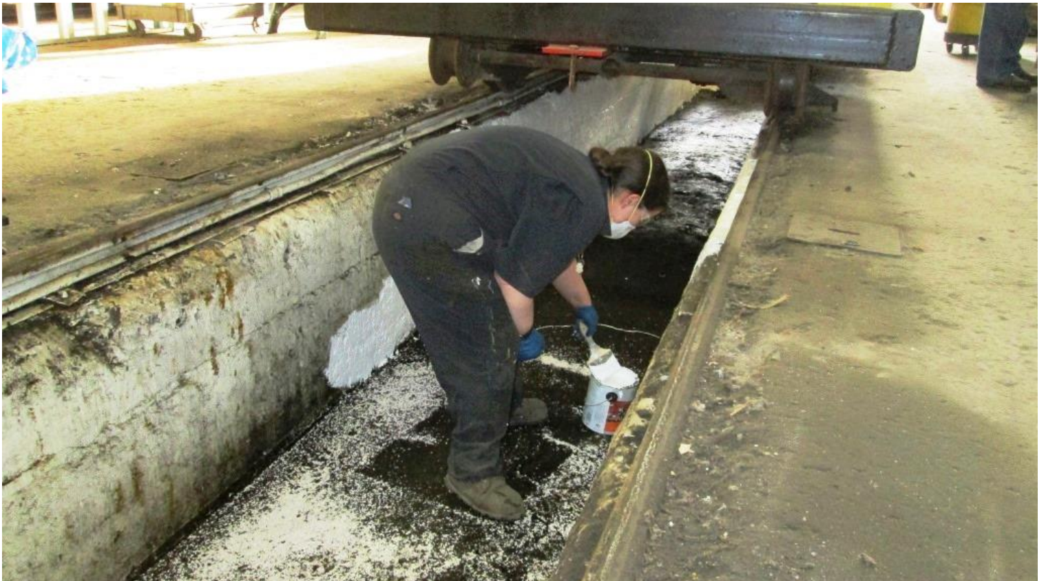
Heather paints the inspection pit at Bay 4 of the Erecting Shop
