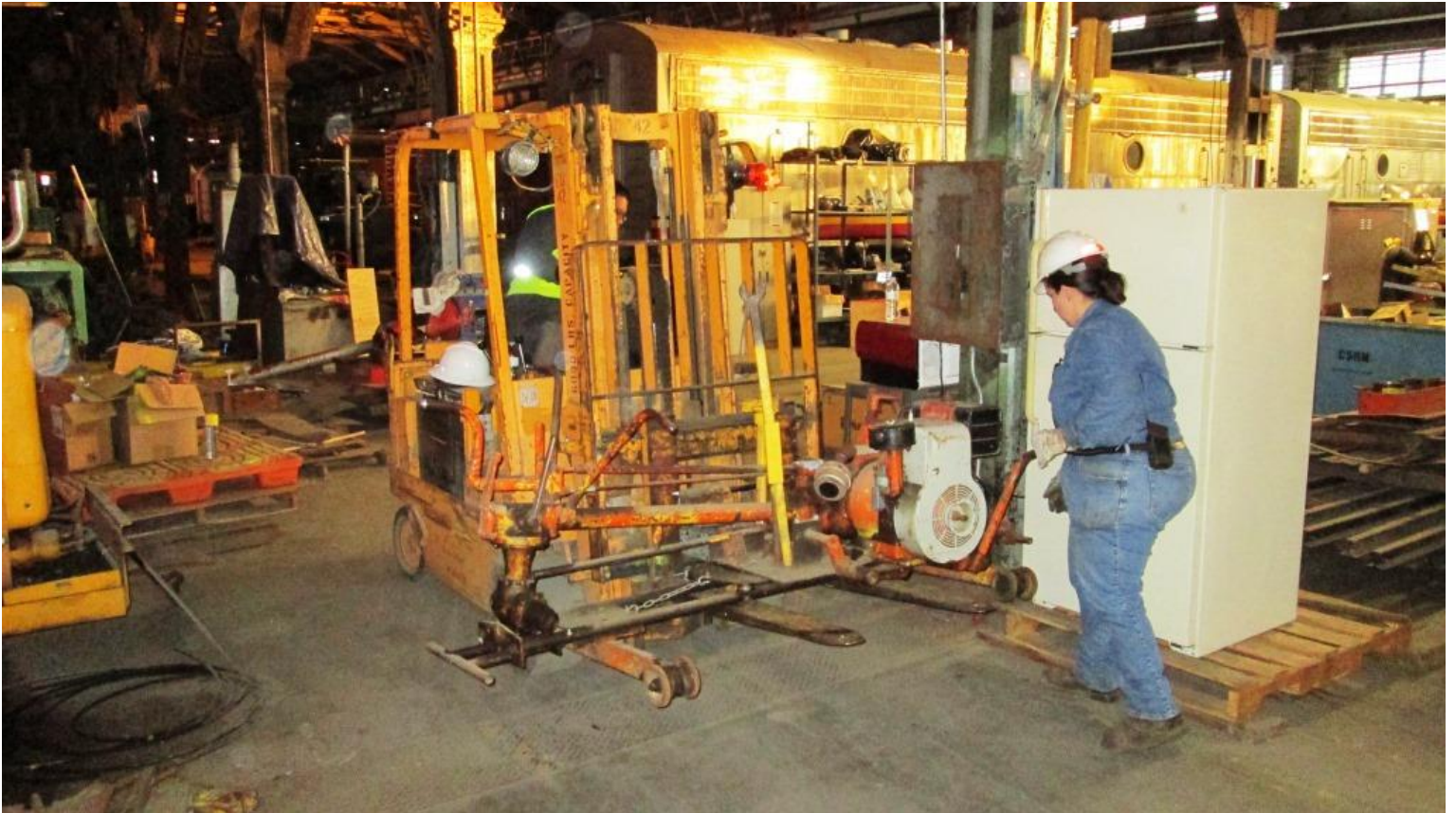
Heather guides Anthony on the forklift carrying a bolt-machine
