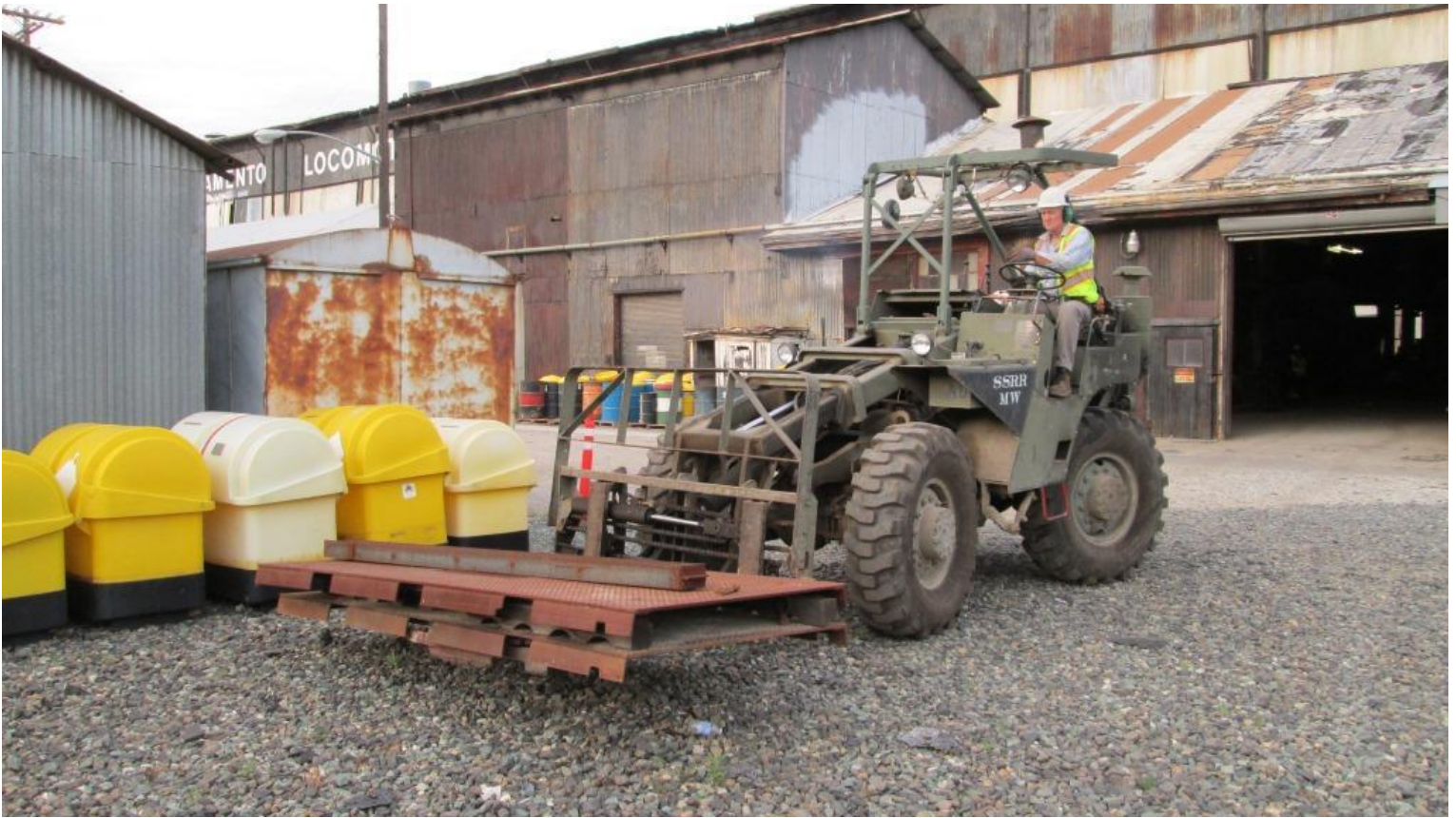
Steve on Big Green re-arranging materials in our materials yard for easier access
