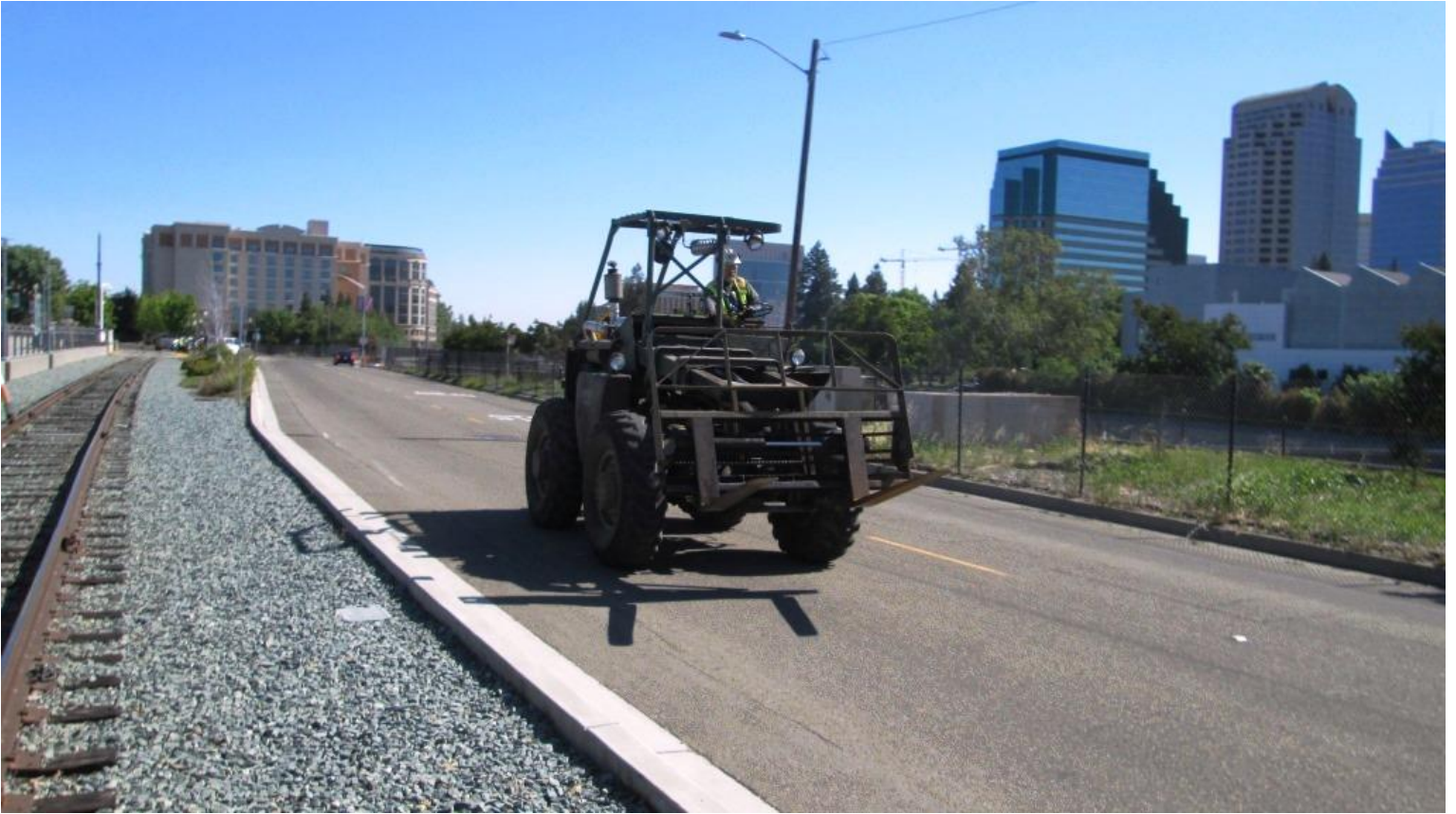
Mike F. on Big Green rushes past the job-site to collect dead-ties at Miller Park
