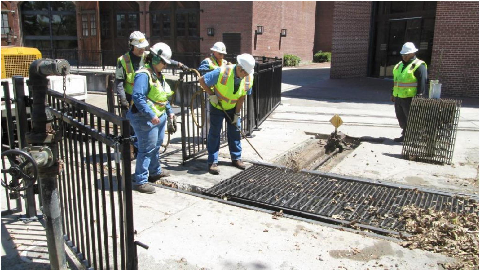
Ed handles the air-wand connected to the rail-mounted air compressor for organic debris removal from Switch 1
