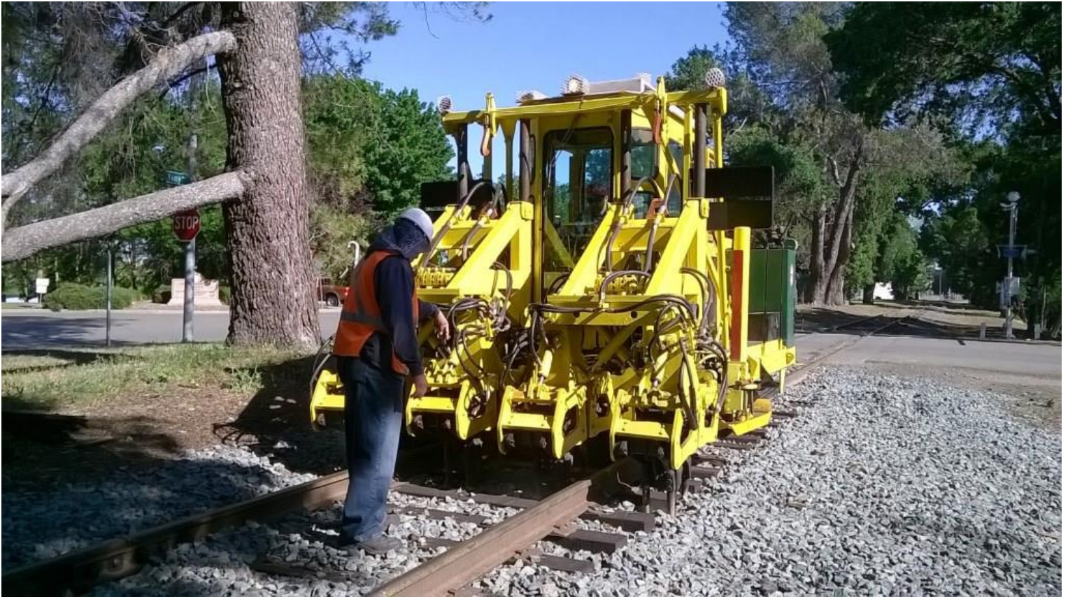
Jose provides guidance from the ground for Chris who is operating the tamper
